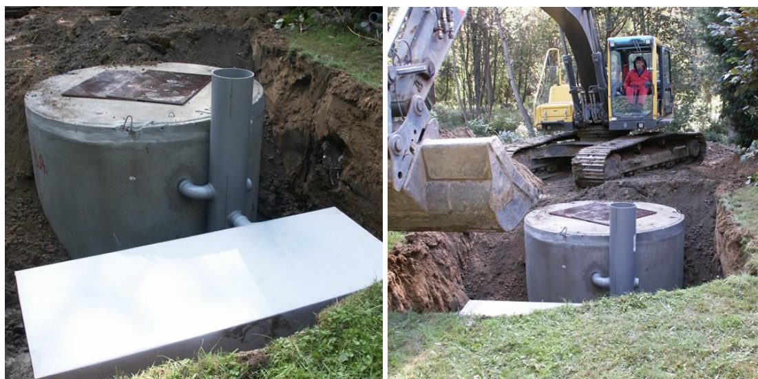
Figure 39. Installation of a BelleAqua SAF 1 - 6 IE with effluent infiltration ( www.belleaqua.be )
