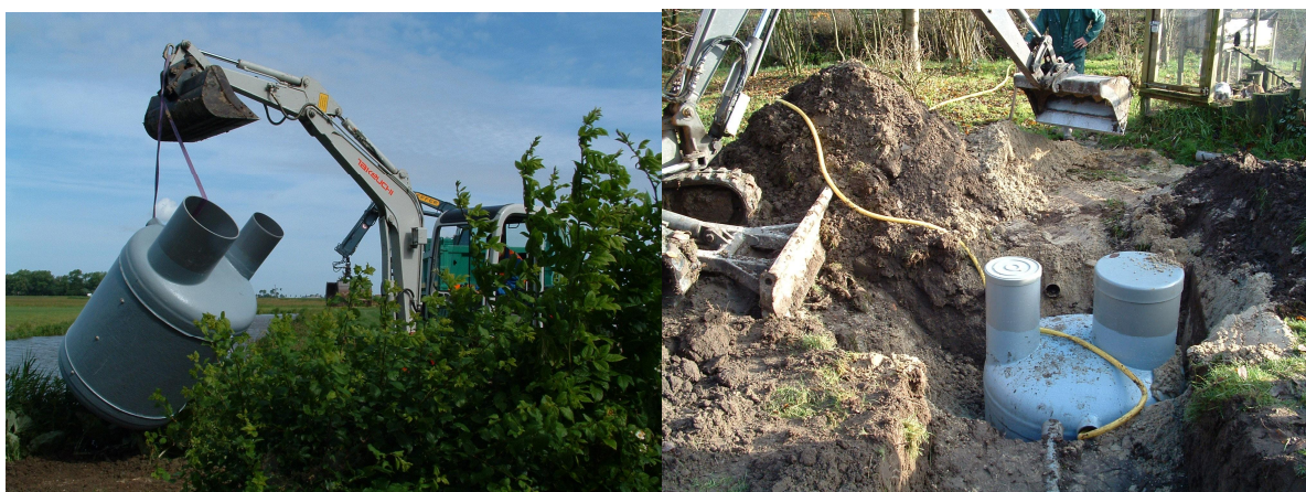
Figure 41. Compact system based on the activated sludge process of Afmittech Friesland
